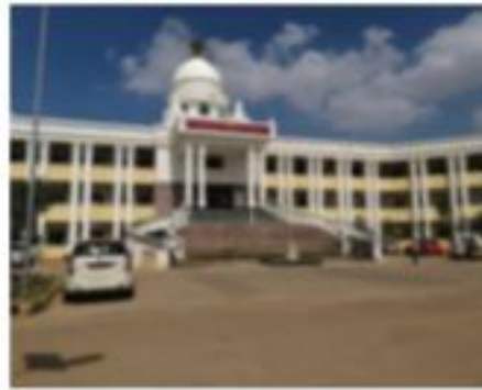
DC OFFICE DEVANAHALLI
