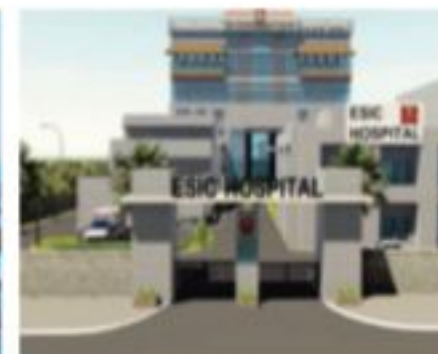
ESI HOSPITAL UNDER CONSTRUCTIONS
